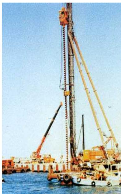
**SANWA AUGER MODEL D-60H USED FOR A SOIL CONSOLIDATION WORK BY INJECTION OF CEMENT SLURRY IN UMMSAID, QATAR**
