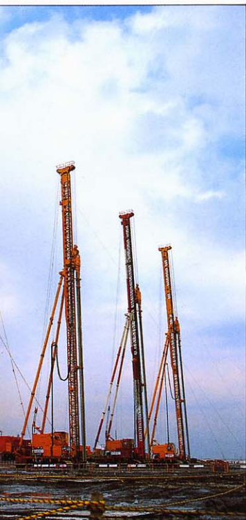
consolidation work ( 2-SHAFTS )
