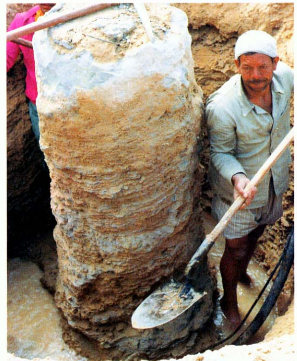
Constructed P.I.P. Pile
