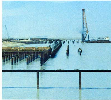
Overall View of the Job Site
