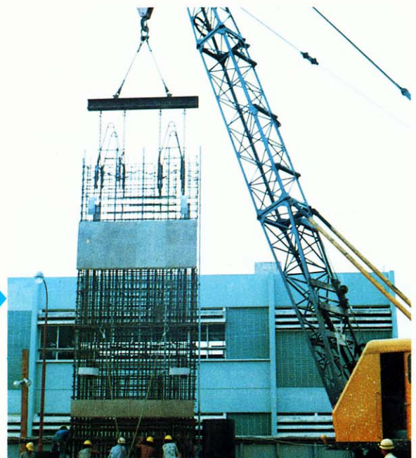
Installing Reinforcement Cage
