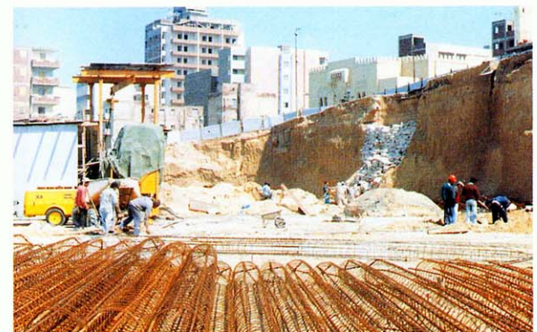
Reinforcing Steel Cage
