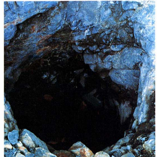
Bored Hole in the boulder layer
