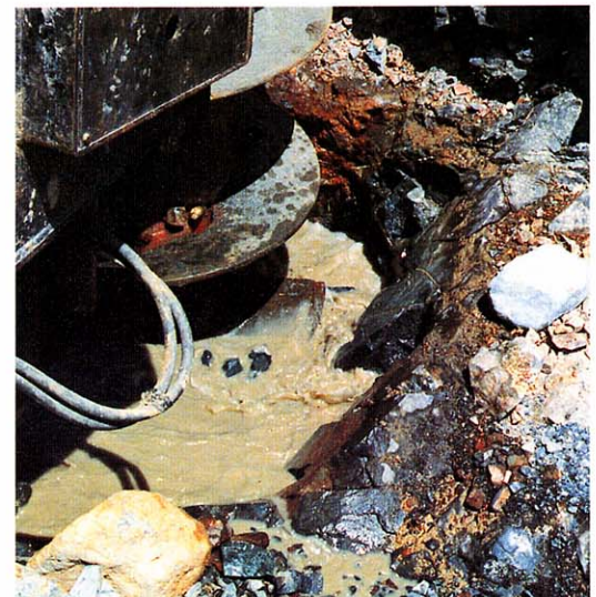
Boring with bentonite solution
